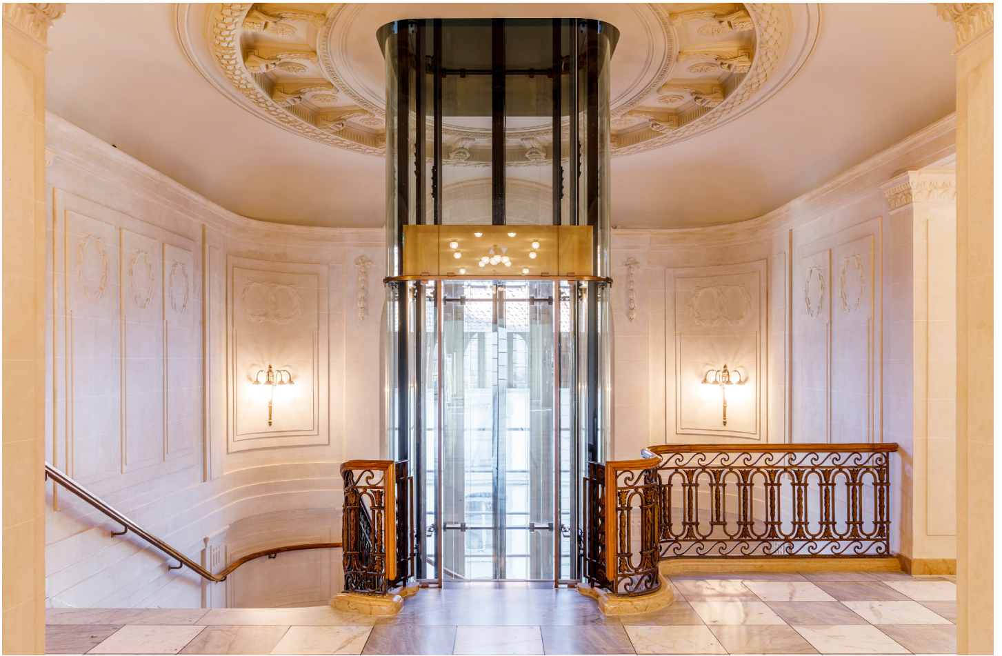
The glass lift shaft pierces the ceiling above the second floor and leads from the public area to the offices.
