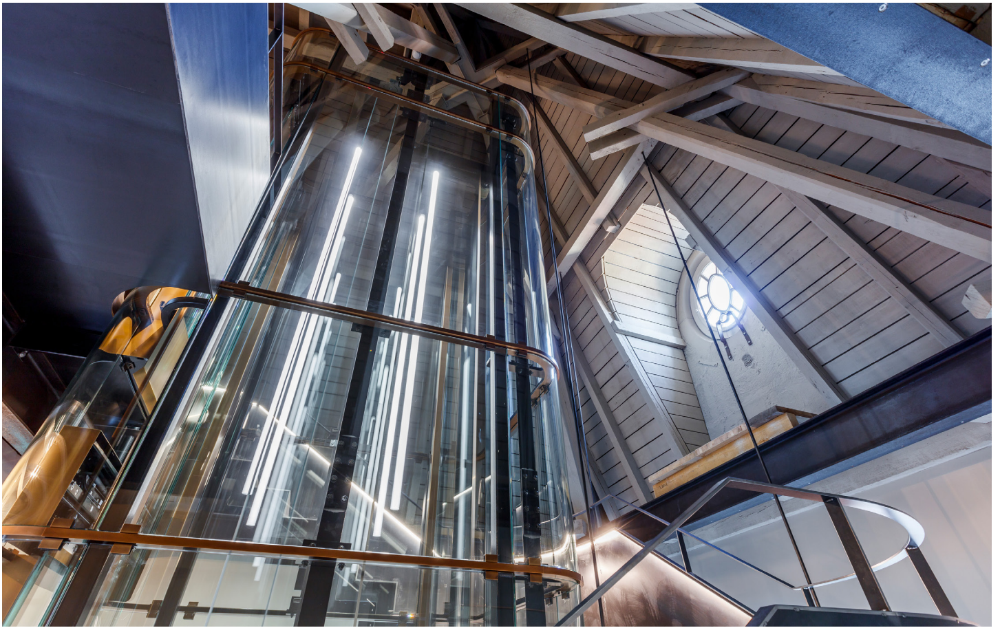
The tight space conditions demanded meticulous planning and execution.
